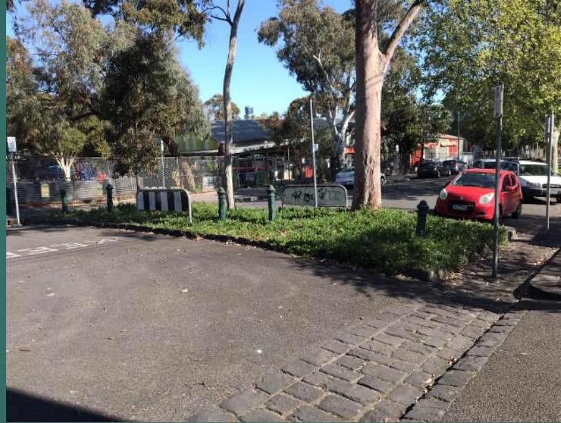
Kerb extensions North Melbourne Primary Melbourne
