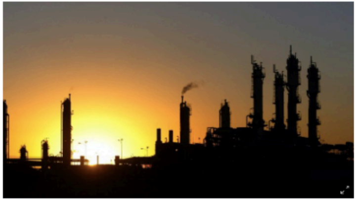
A natural gas plant in the Cooper Basin. BRENDAN ESPOSITO
